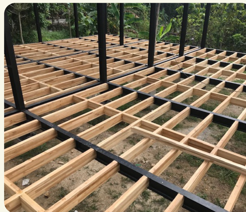
Steel H-Beams 150 + Recycled Teak Glulam Substructure
