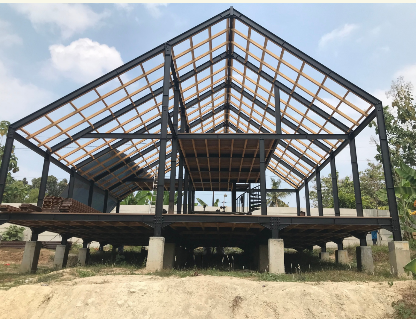
Steel H-Beams 150 + Recycled Teak Glulam Substructure
